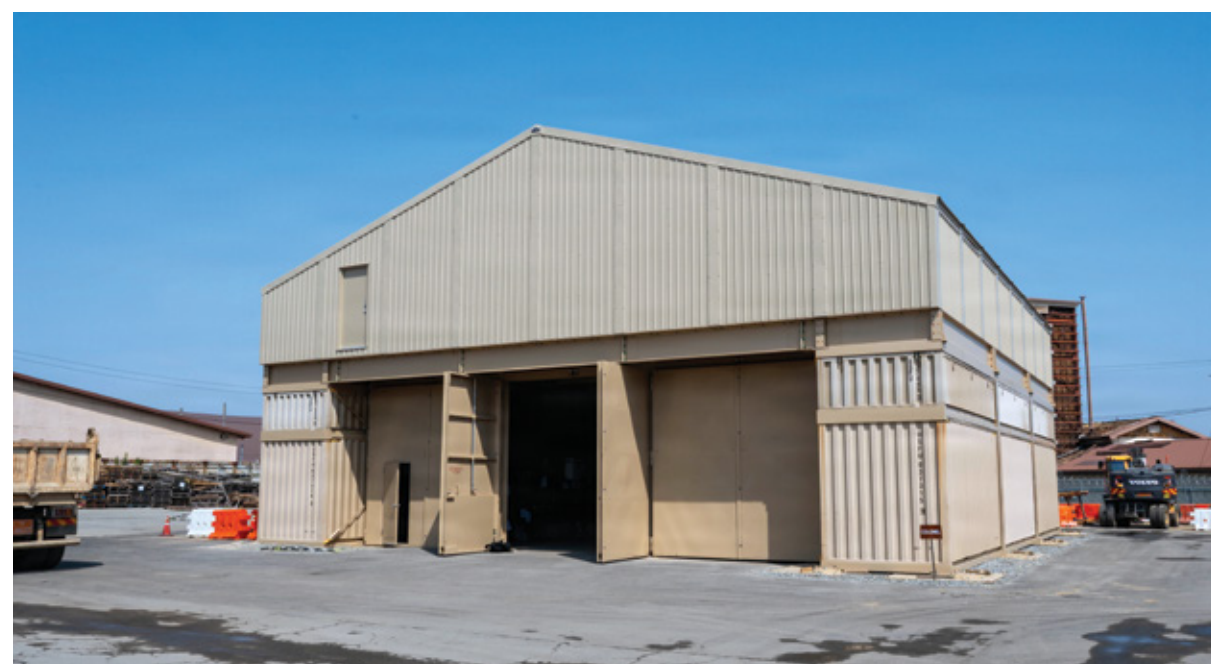
The 51st Civil Engineer Squadron, in coordination with the 51st Logistics Readiness Squadron, completed construction of the only expeditionary storage and protection facility on the Korean Peninsula at Osan Air Base, Republic of Korea, April 27, 2026. The ESAP facility is a hardened, modular structure that provides protected storage for critical equipment while enhancing the base's readiness and ability to operate in contested environments. ▲
