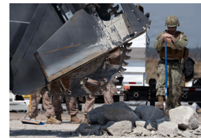
A wheel saw is used during a joint-service Rapid Damage Repair training at Kunsan Air Base, Republic of Korea, March 23, 2026. RDR encompasses all actions required to quickly repair runways to recover operations on an airfield after an attack. RDR may be conducted during conditions such as inclement weather, chemical, biological, radiological, and degraded environments. ▲
