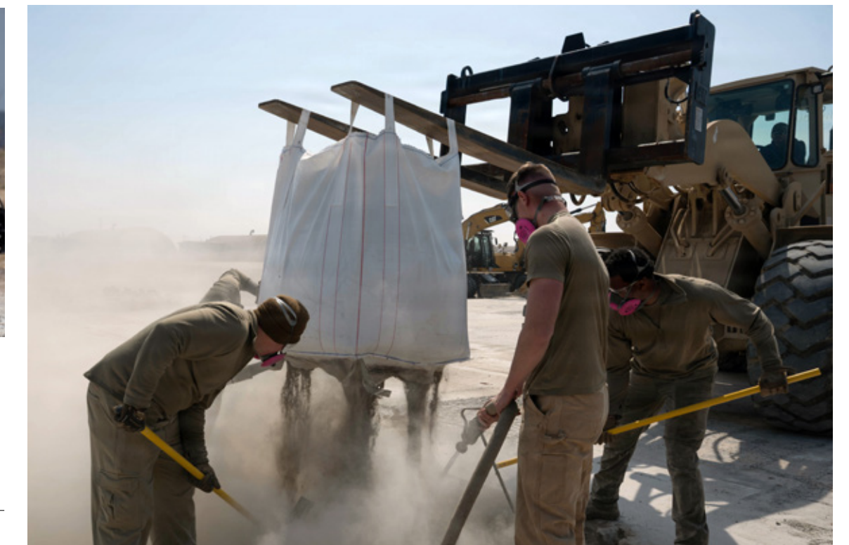
A wheel saw is used during a joint-service Rapid Damage Repair training at Kunsan Air Base, Republic of Korea, March 23, 2026. RDR encompasses all actions required to quickly repair runways to recover operations on an airfield after an attack. RDR may be conducted during conditions such as inclement weather, chemical, biological, radiological, and degraded environments. ▲
