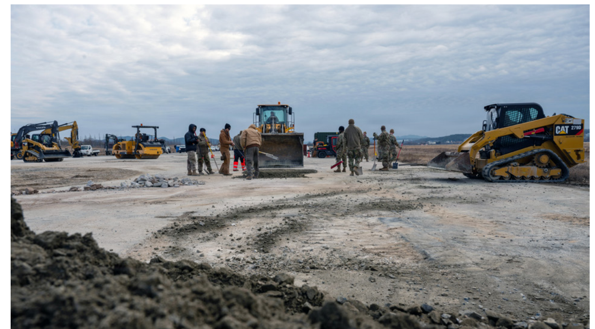
U.S. Air Force Airmen assigned to the 51st Civil Engineer Squadron remove excess debris during Rapid Osan Airfield Recovery training at Osan Air Base, Republic of Korea, Feb. 27, 2026. The panel-based technique is designed to rapidly return the runway to operational status in support of aircraft launch operations. ▲
