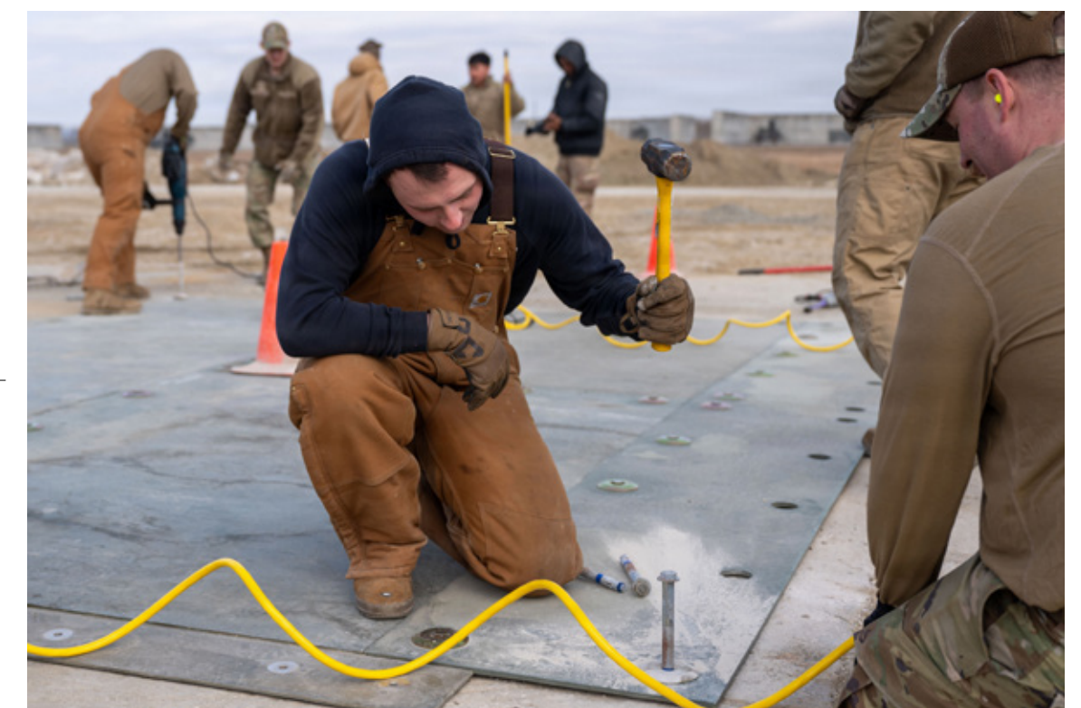
U.S. Air Force Airmen assigned to the 51st Civil Engineer Squadron remove excess debris during Rapid Osan Airfield Recovery training at Osan Air Base, Republic of Korea, Feb. 27, 2026. The panel-based technique is designed to rapidly return the runway to operational status in support of aircraft launch operations. ▲
