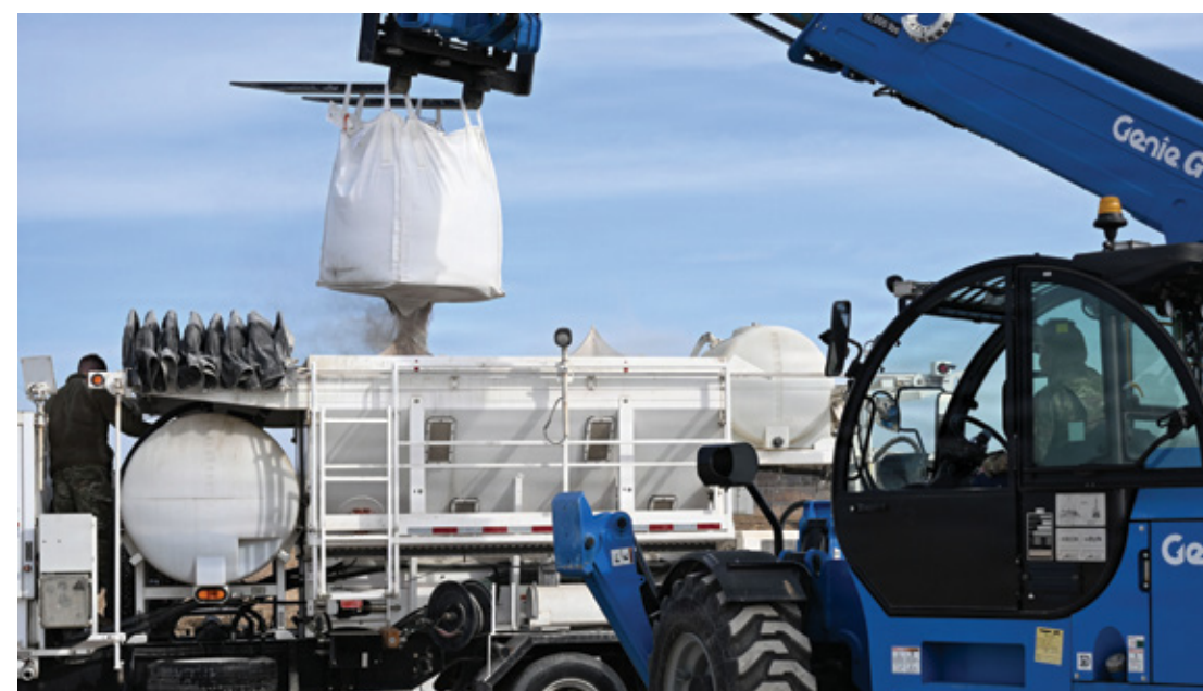
U.S. Air Force Airmen assigned to the 51st Civil Engineer Squadron mix concrete powder and water in a volumetric mixer during Rapid Osan Airfield Recovery training at Osan Air Base, Republic of Korea, Feb. 26, 2026. The training evaluated ROAR, an installation-specific method focused on restoring minimum runway capability quickly during contingency operations. ▲
